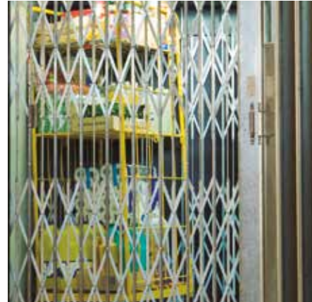
Lift car folding doors: manual picket gates
