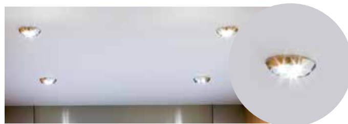
Ceiling with LED spots
